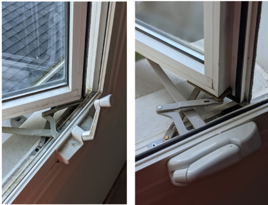
New window hardware, before & after
